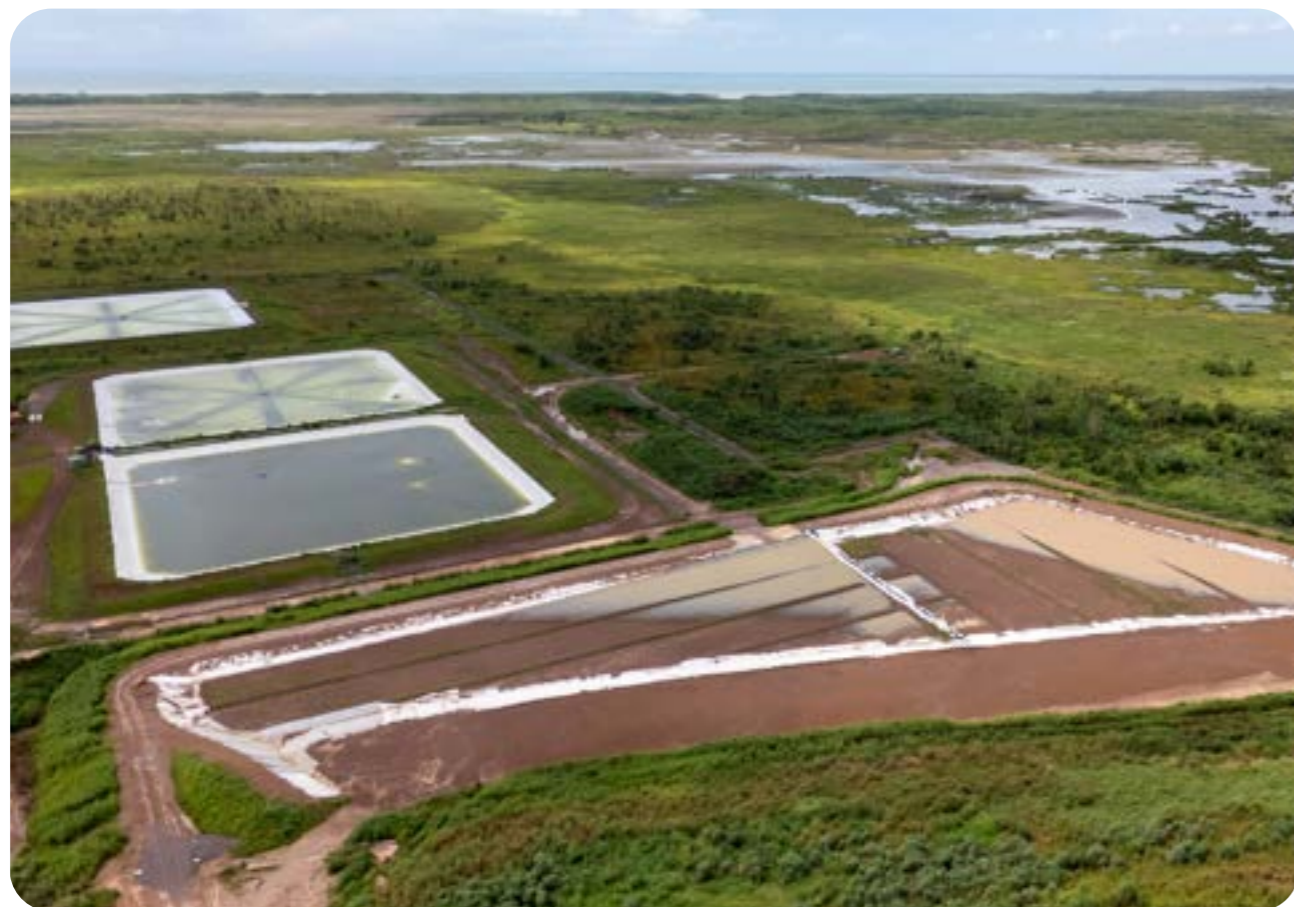
Shoal Bay Waste Management Facility – Stage 2 northern expansion
