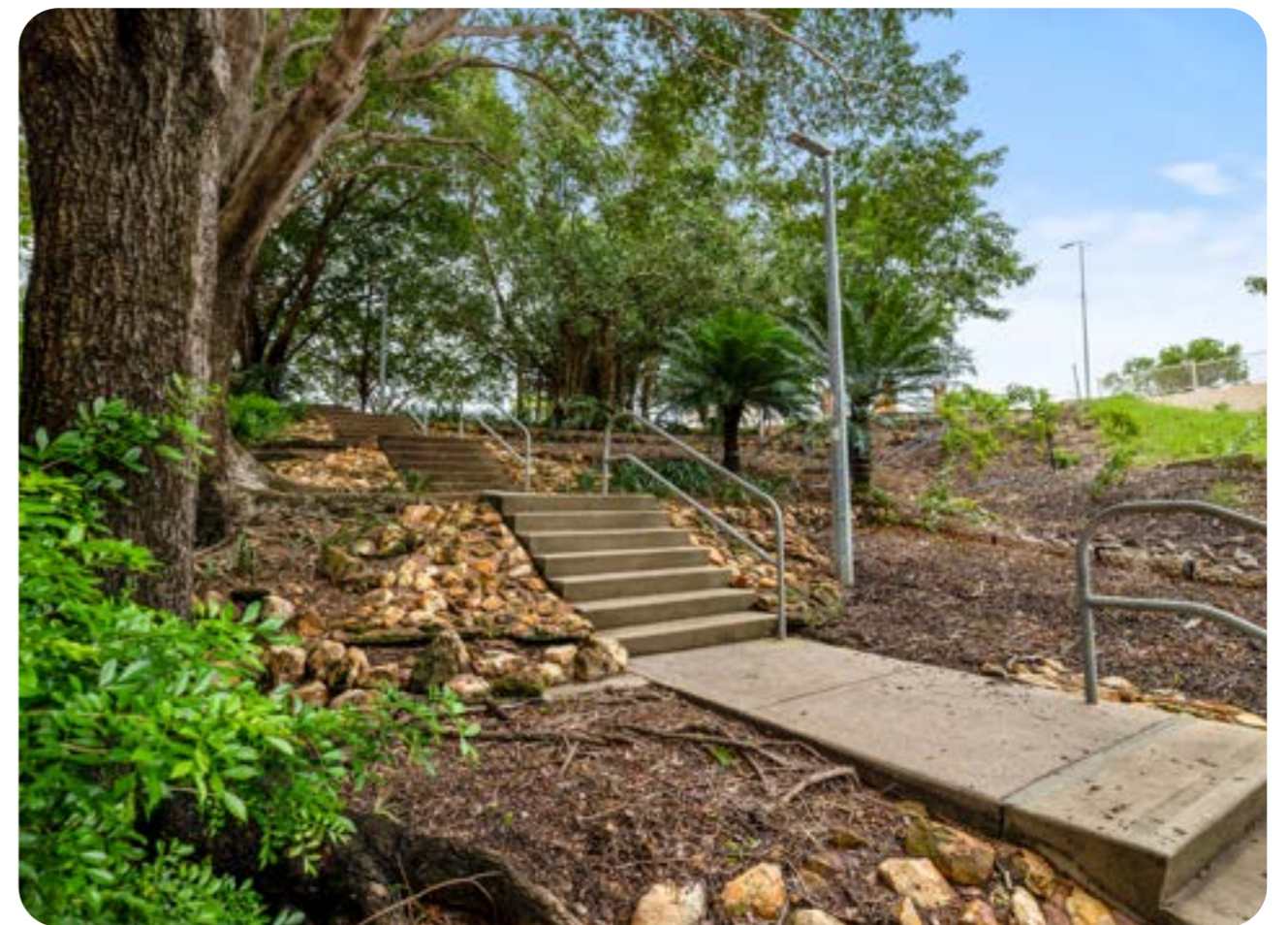
Travellers Walk landscaping upgrades
