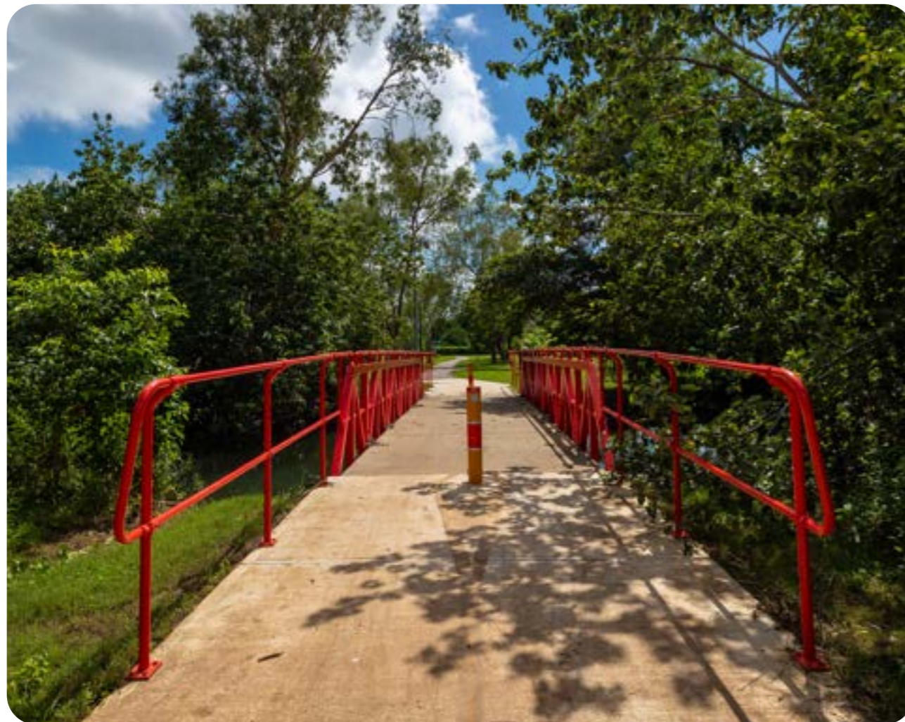
Jingili Water Gardens footbridge upgrade
