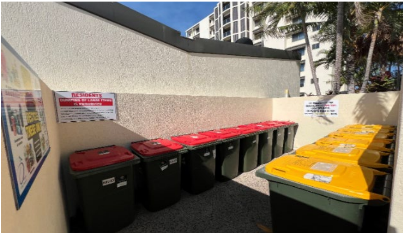
Figure 6: Example of manual service bin storage area
