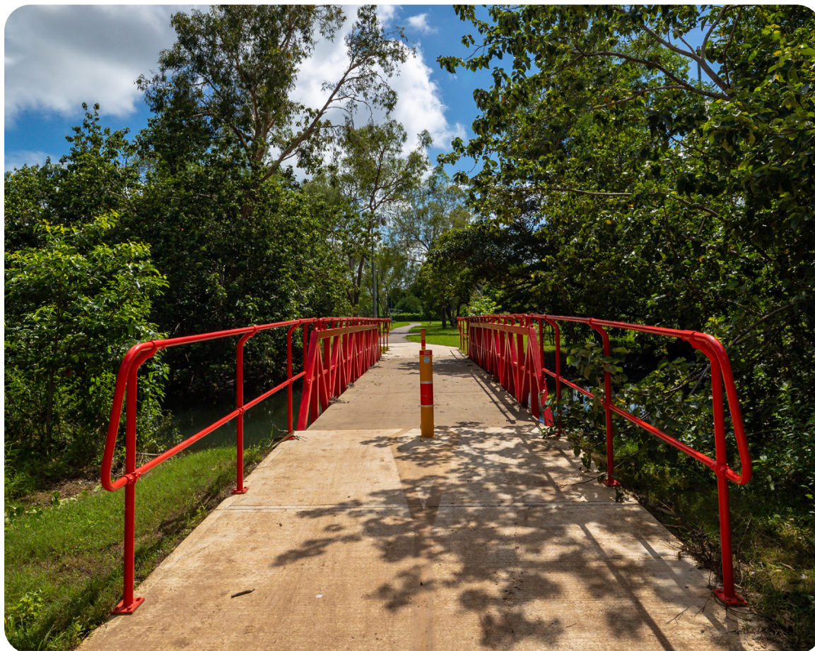
Jingili Water Gardens footbridge upgrade
