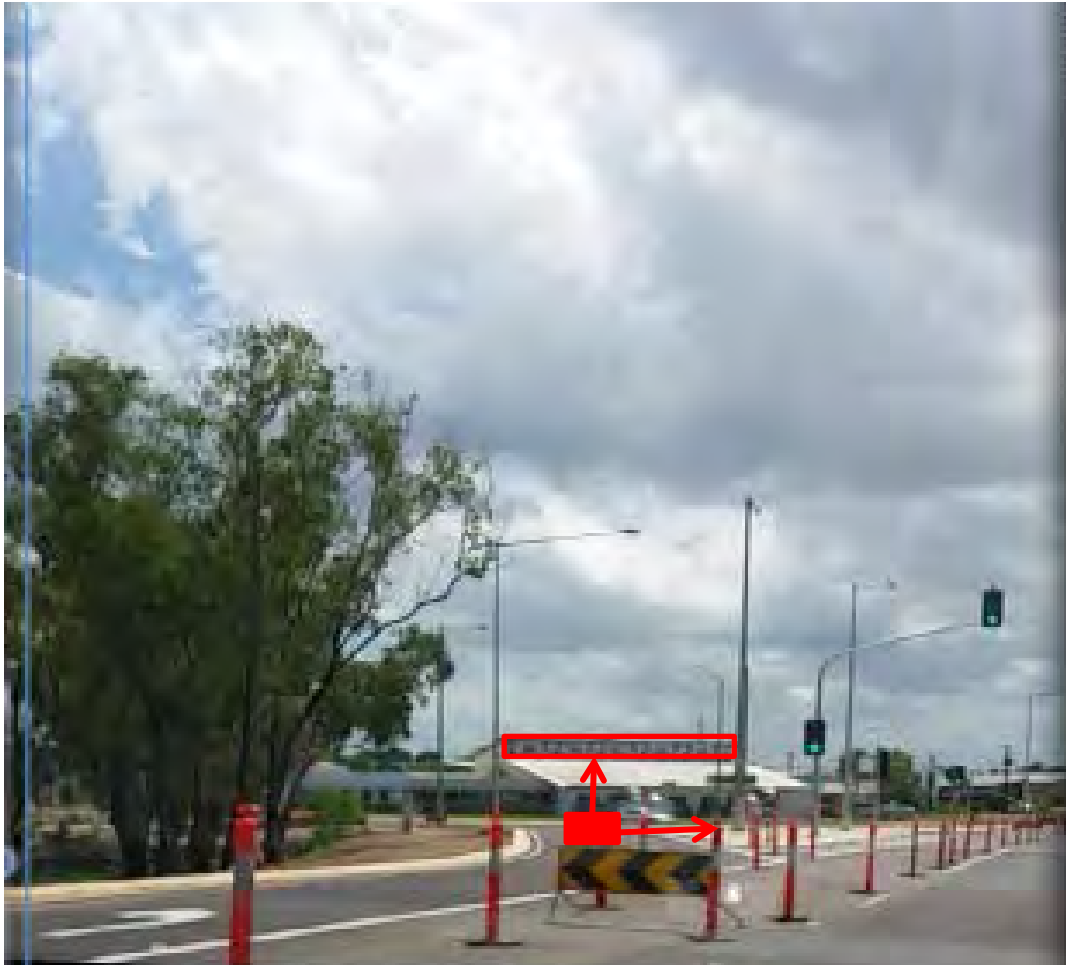
VEHICLE ENTERING BENISON - YIELD ON LEFT TURN OFF TBD : POSSIBLE DISTRACTION DUE TO SIGN PLACEMENT.
