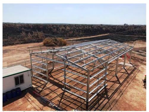
Image 1: Construction of the site shed which will house the process tanks
