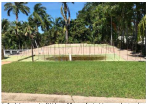
Figure 3 - Roof of garage at Lot 5390 Lambell Terrace. Steel reinforcement has been installed in preparation for construction. (13/07/2017)
