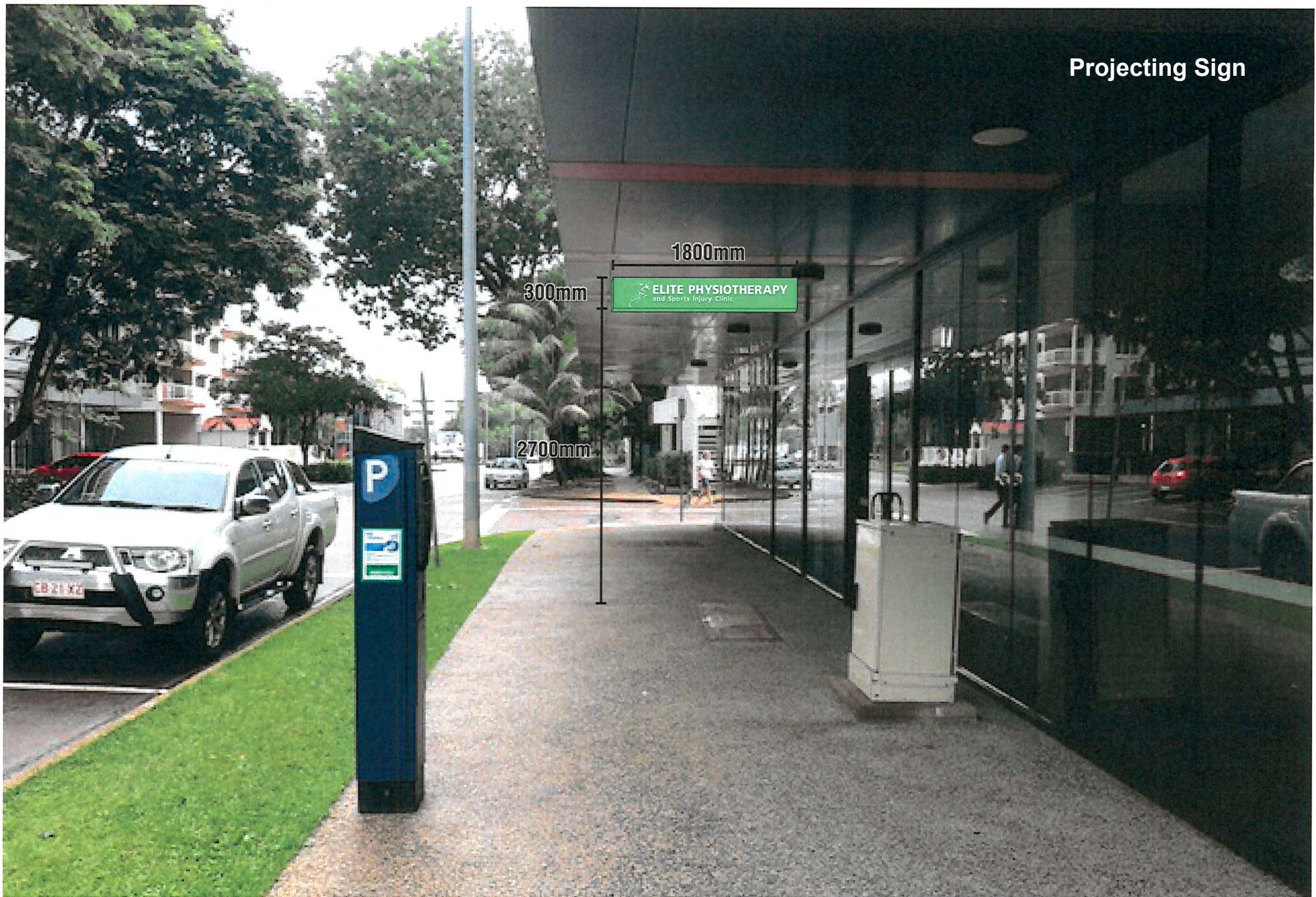
X1 DOUBLE SIDED LIGHTBOX @ 1800mmW x 300mmH INSTALLED HARD AGAINST THE SOFFIT, 2700mm FROM GROUND LEVEL TO THE BOTTOM OF THE LIGHT BOX
