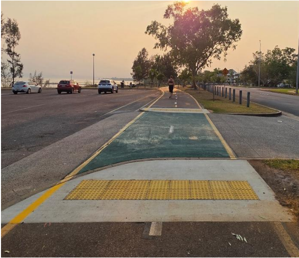
Tactile Indicators at Nightcliff Foreshore
