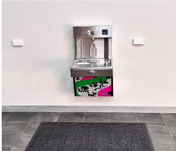
Casuarina Library: Installation of accessible water bubbler
