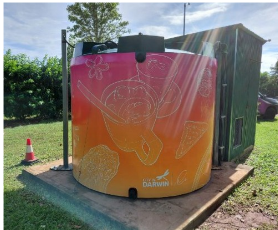
Replaced irrigation tank.
