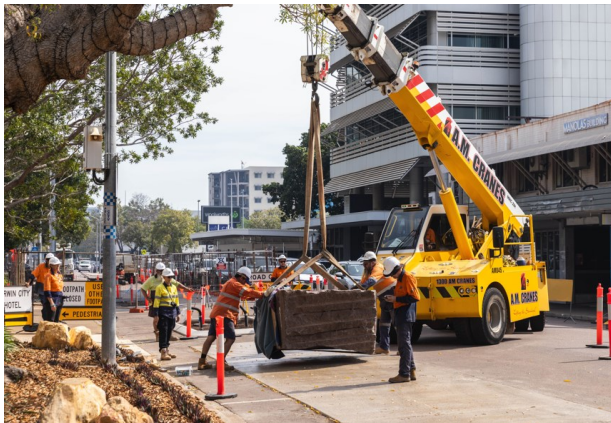
Install – Foundation Stone
