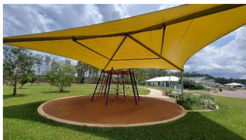
Mirawood Park Facilities
