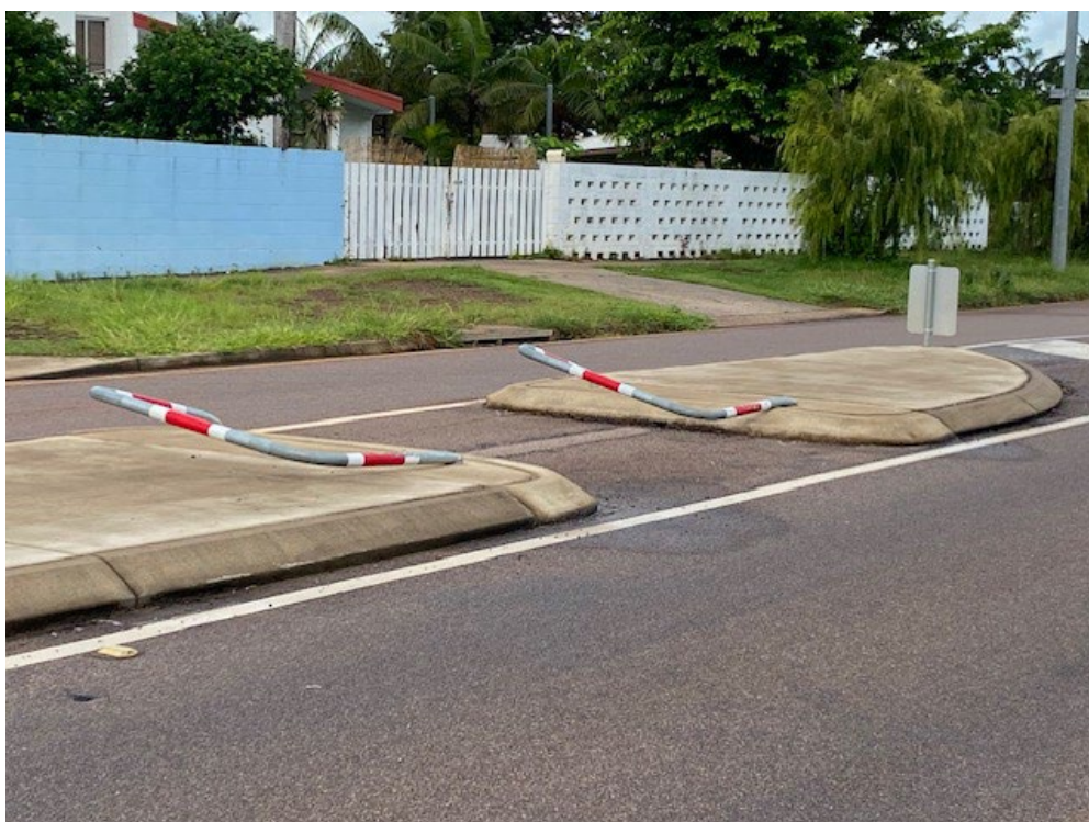
Figure 2: Knocked over safety bollards on Nightcliff Road near Chapman Road. These have been hit and damaged twice within 18 months.
