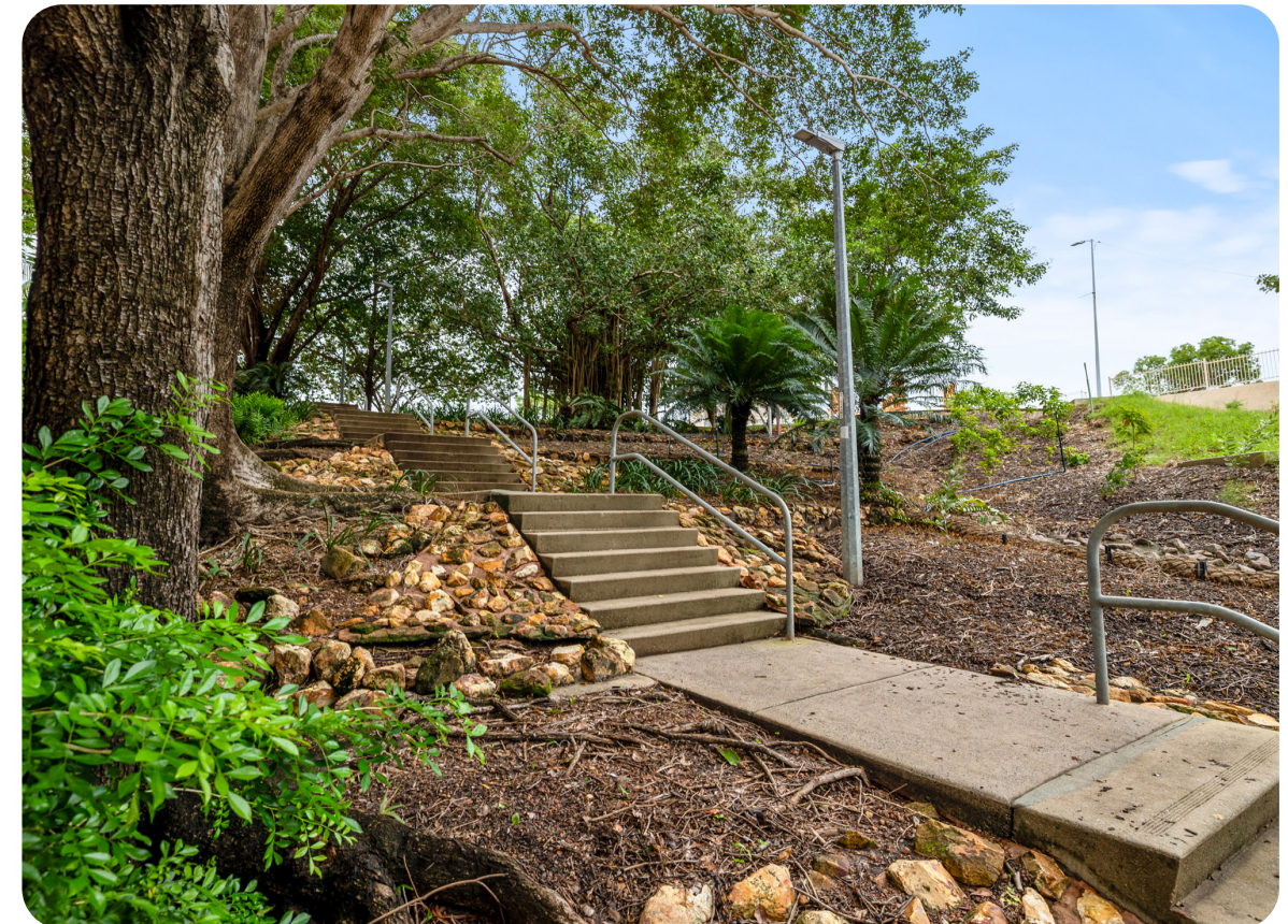
Travellers Walk landscaping upgrades
