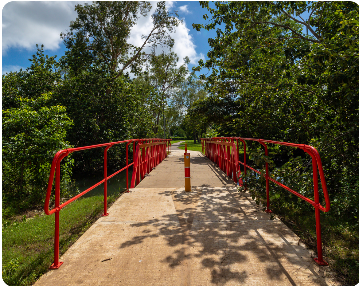
Jingili Water Gardens footbridge upgrade
