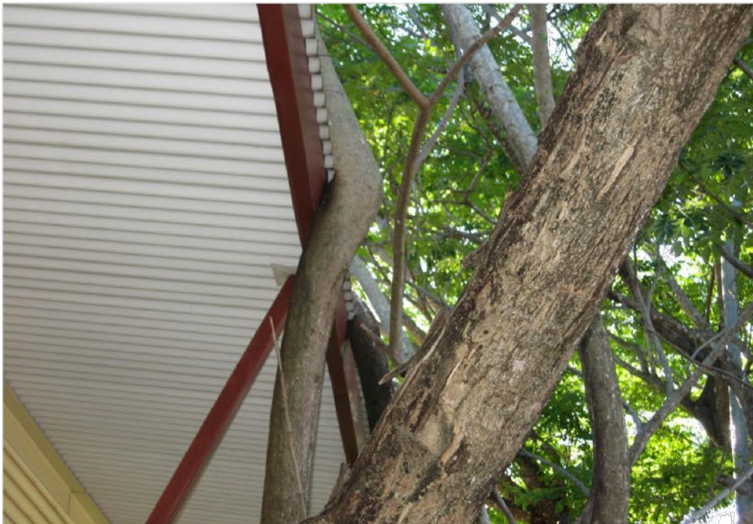
Photo # 13 showing Raintree damaging a roof.
