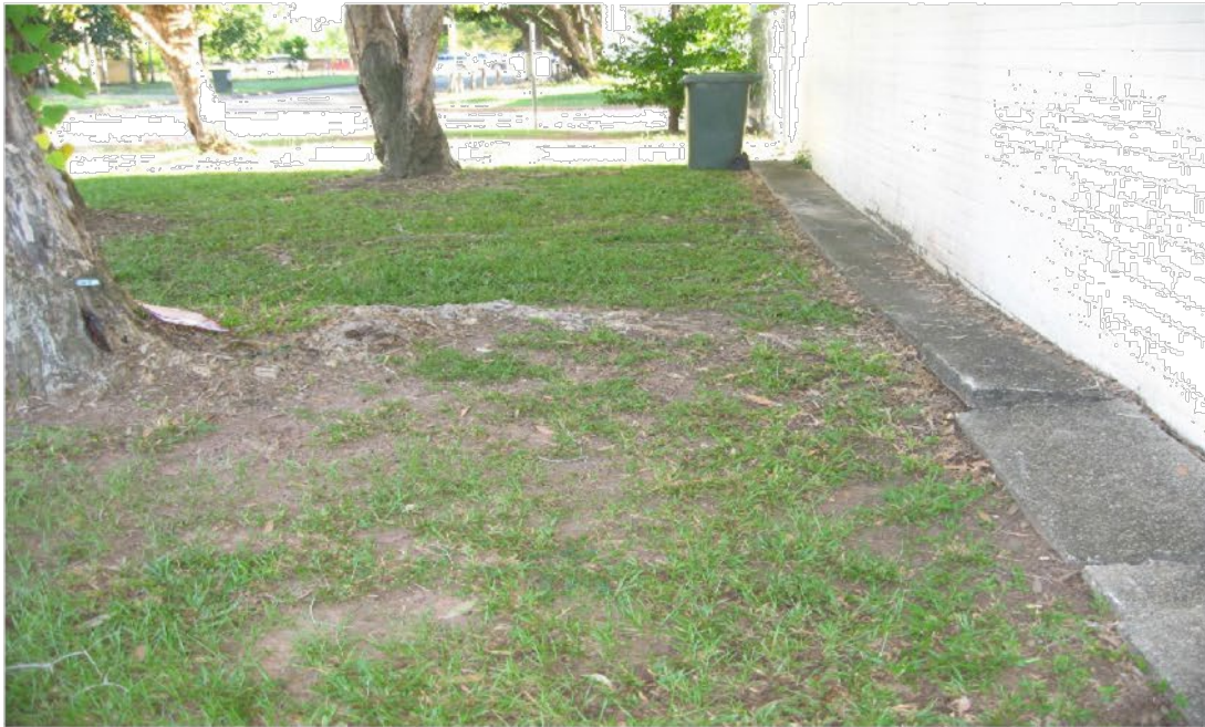
Photo # 14 showing roots from a Melaleuca damaging infrastructure.
