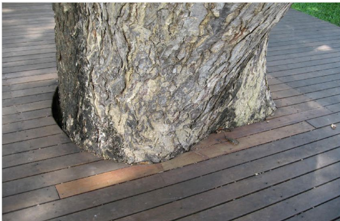
Photo # 9 showing a landscaper's best effort to kill a Raintree or destroy the deck. The tree was given a new lease of life by making the hole bigger.
