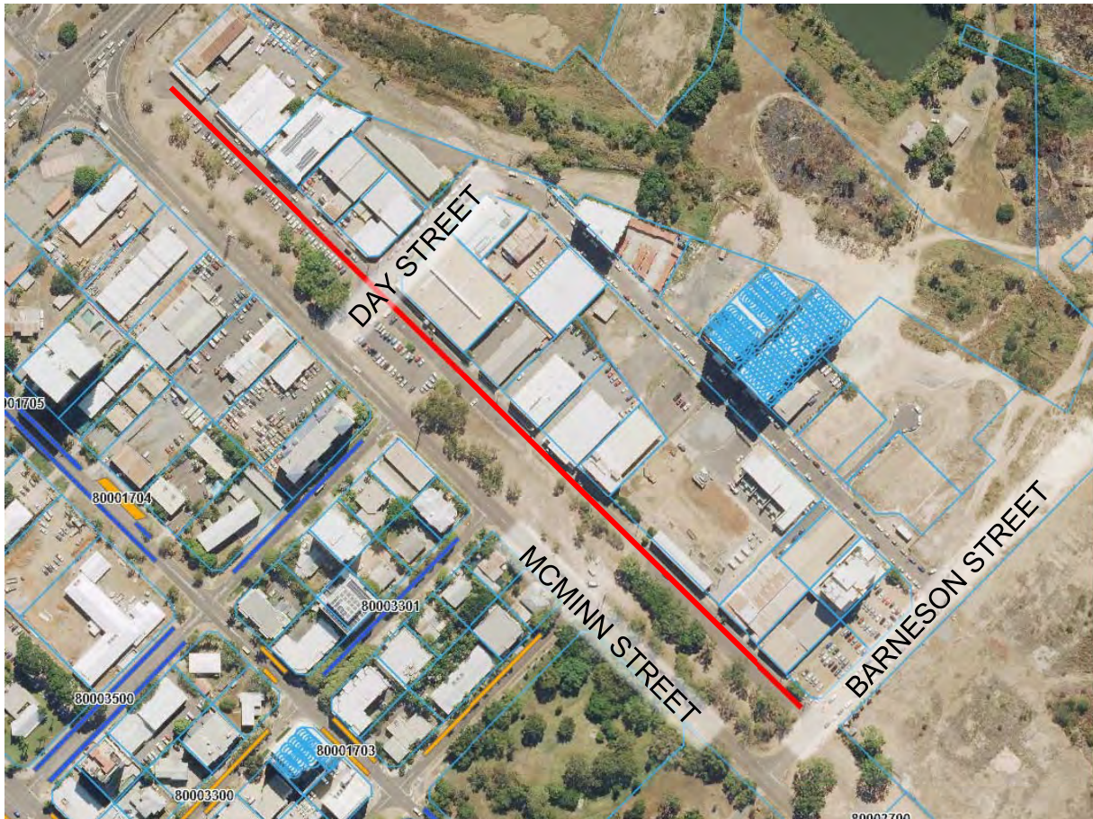
Image 1: Aerial of McMinn Street and Service Road (Red)
