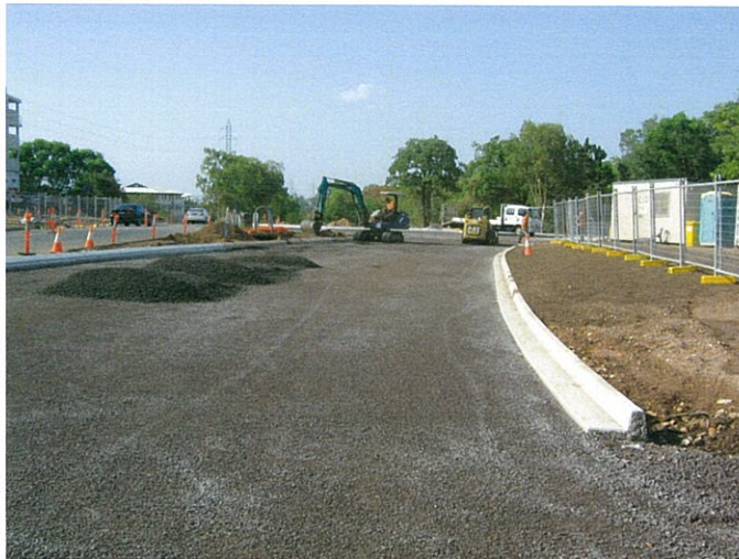
Construction of Northern Approach to New Roundabout - New Kerbing And Road Base
