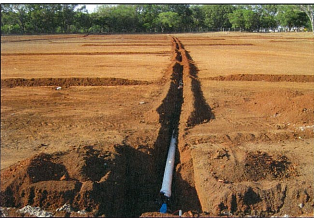
3. Irrigation in subgrade.
