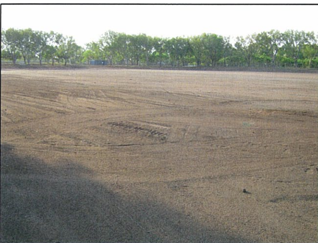
5. Final treatment of top soil ready for hydromulch seeding.
