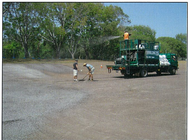
6. Hydromulching seed onto final surface level.
