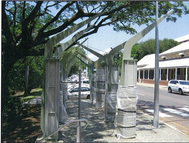
Figure 3. View of blade installation at Area 1 with stainless cables, the Waterfront walkway entrance.
