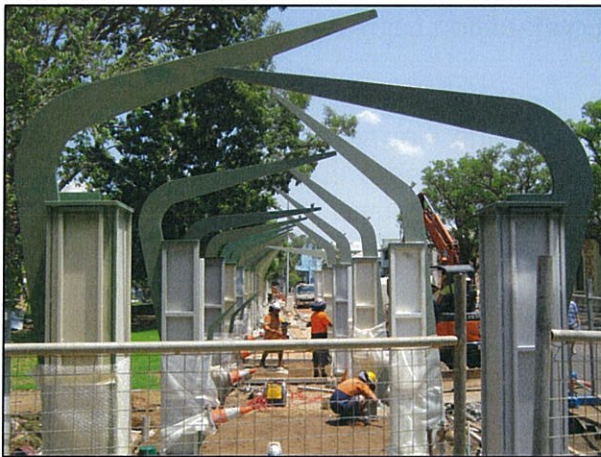
Figure 1. Installation of blade structures at Northern end of site, Area 4.
