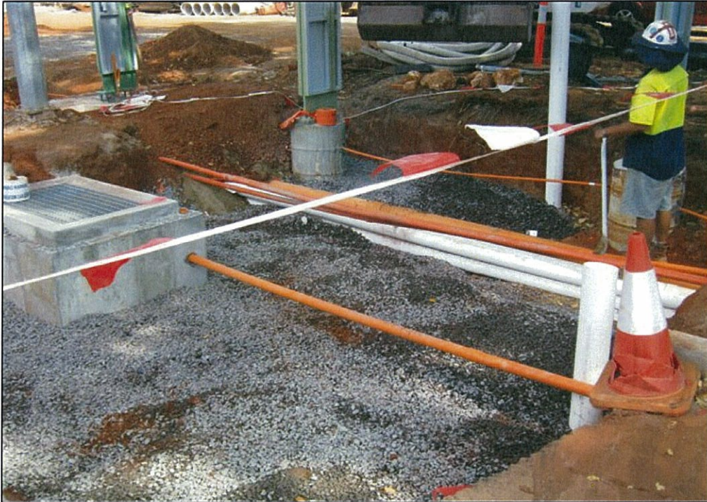
Extent of tree pit showing stormwater over flow, services and drainage layer
