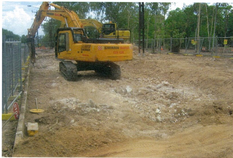
Rock Breaker Excavating the Stormwater Drain
