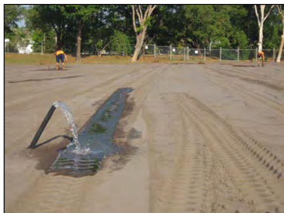
Photo 4. Locating irrigation risers for installation of sprinkler heads.
