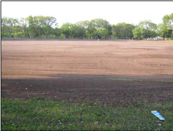
Photo 3. Top soil final treatment, ready for grassing.
