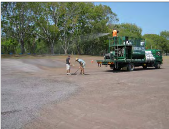
Photo 5. Hydromulching of seed, paper mulch and tacifier commences 12 October 2009.
