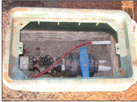
Photo 2. Typical irrigation dry box set on pavers with isolation valve and solenoid.
