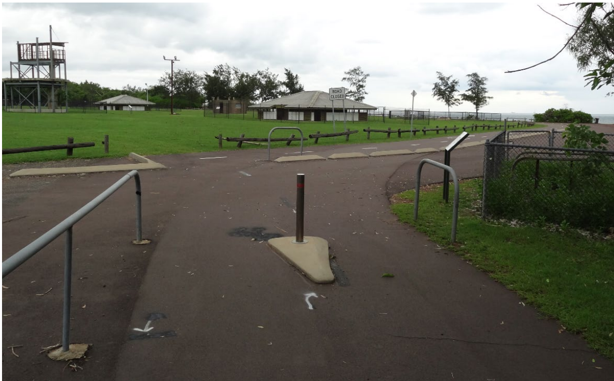
Example of poorly located handrail at a path termination
