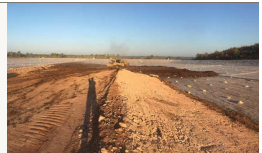
IMAGE 31 Shoal Bay Waste Management Facility - Cell 5
